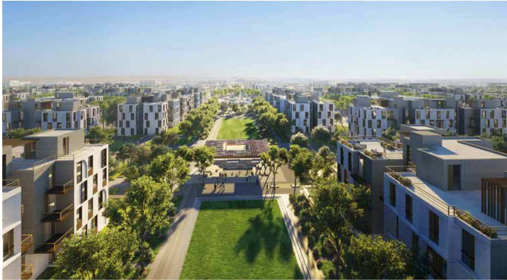
Vye New Zayed Cairo, Egypt
