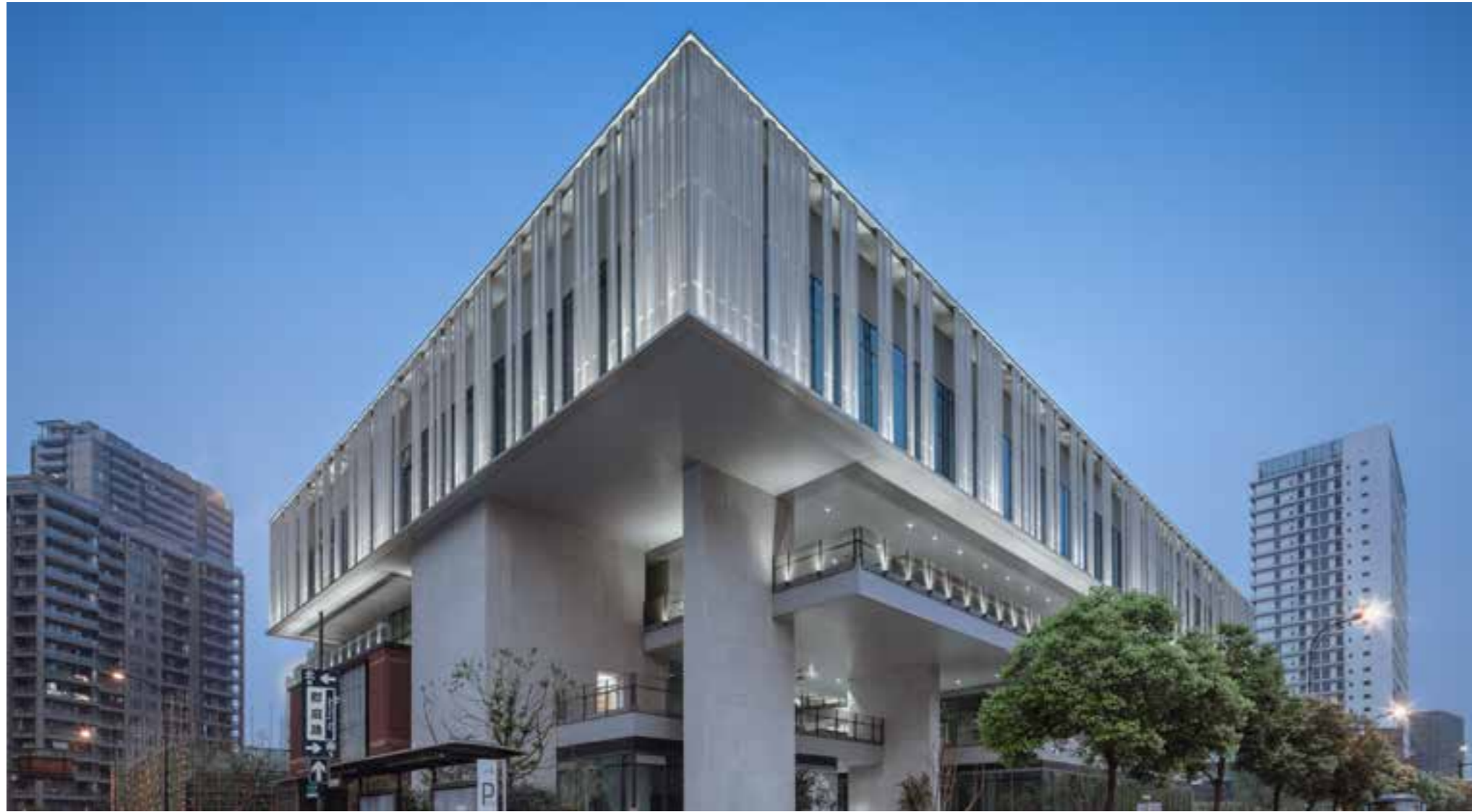
Hangzhou Canal Arts Center Hangzhou, China
