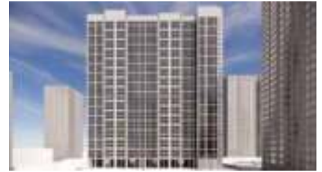
Façade articulation is used to visually group some windows together, creating a diverse fenestration without impacting the built structure
