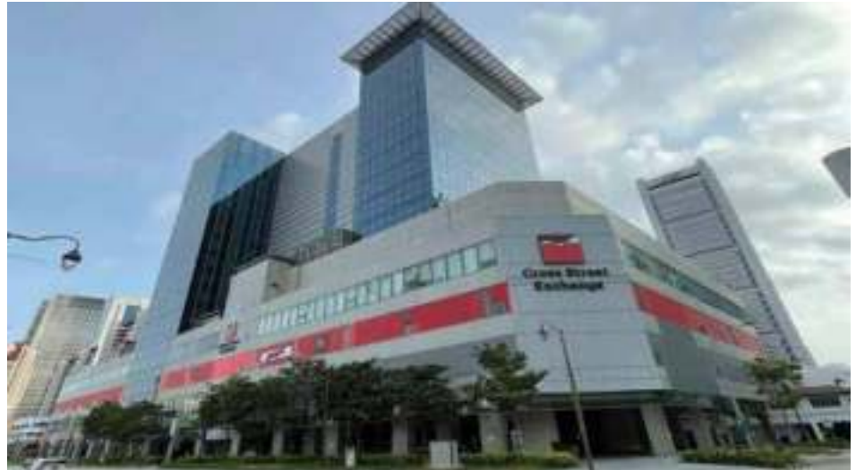
Cross Street, Singapore located on the edge of China Town and the Central Business District – before redevelopment
