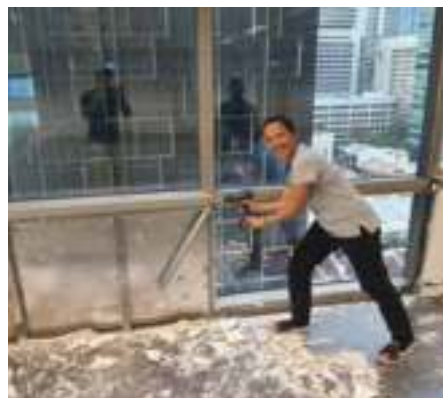
The solid parapet panels were removed to achieve floor-to-ceiling clear-glazed windows
