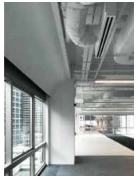
Exposed ceilings were used to increase floor heights
