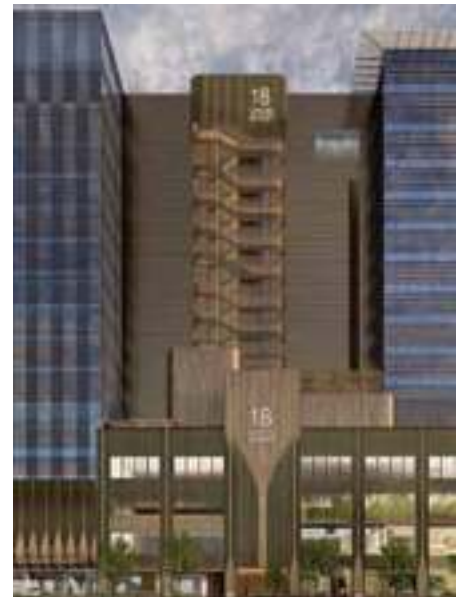
The newly added fire staircase integrates the tower and the podium
