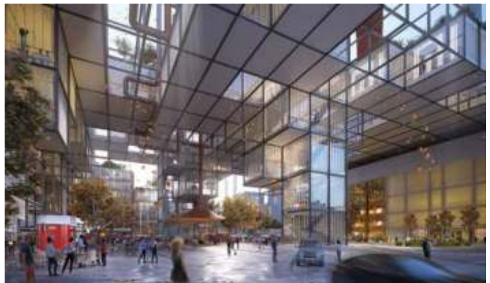
The extension of the industrial steel truss of the powerstation creates a large semi outdoor plaza with a functional office floor and amenities above
